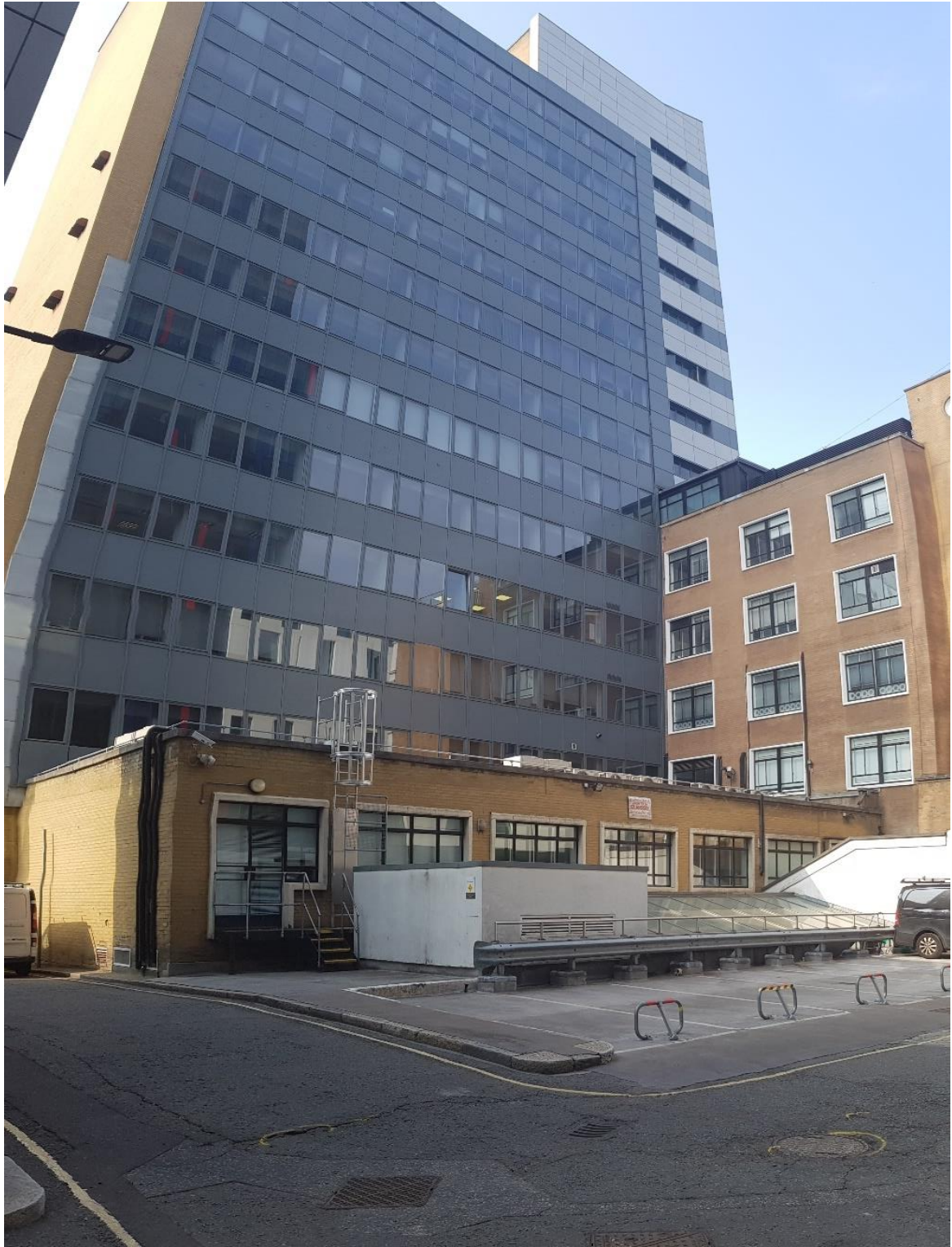
Figure 3: View from St Clare Street towards southwest (Application site)
