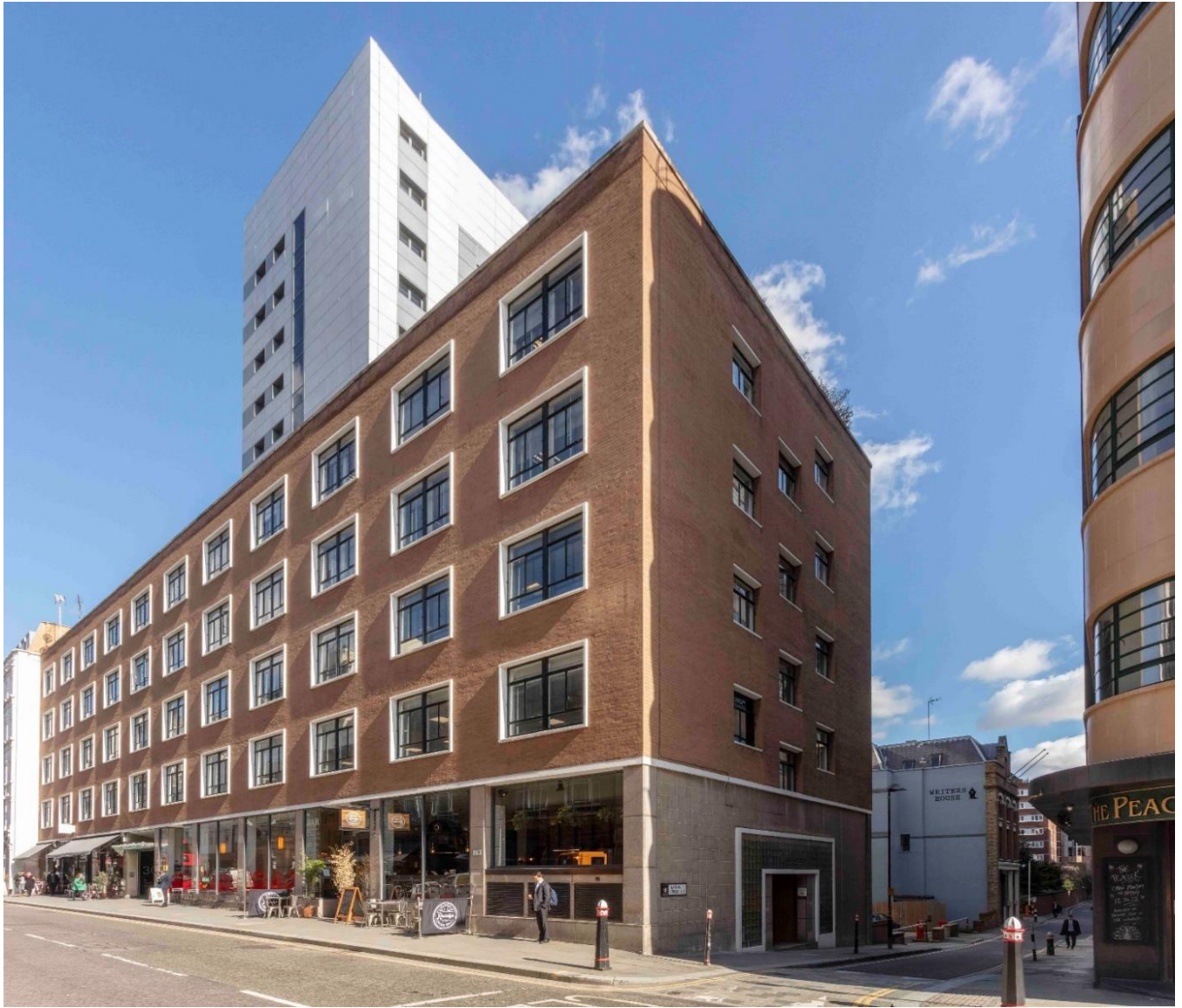
Figure 1: View from Minories towards northeast (Application site)
